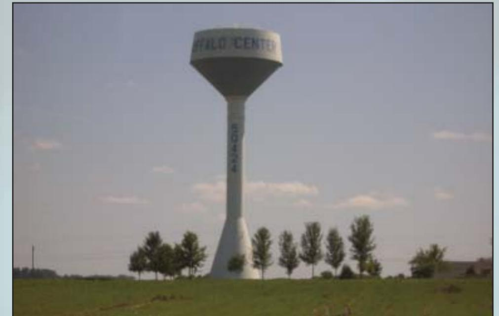
Buffalo Center is a community of about 1,500 people in northern Iowa. The city’s water and wastewater needs are served by a system that includes a water plant with two well heads, chemical feed, filtration and two high service pumps; one elevated tank; and two wastewater lift stations.
